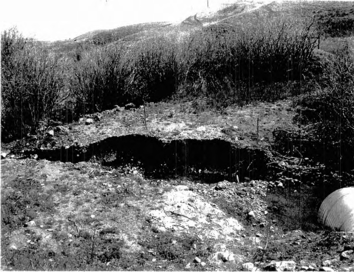
View to the southeast showing remediated area just below culvert. Note that vegetation on both banks (north and south) is beginning to fill in where topsoils were replaced after the excavation and bank reconstruction. Also note the stream cuts beginning to develop.
