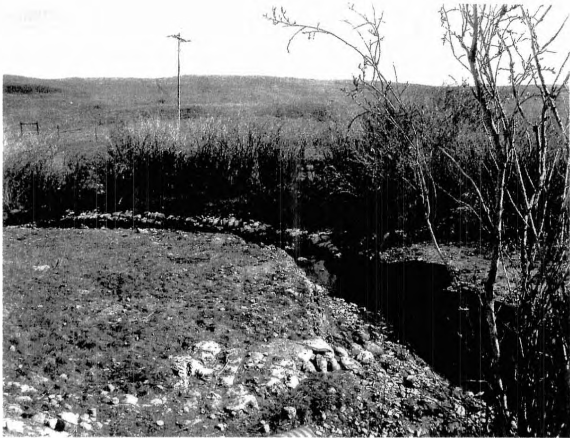
View to the east showing remediation area just east of the culvert. Note that vegetation is filling in on the north bank after the excavation and bank reconstruction.
